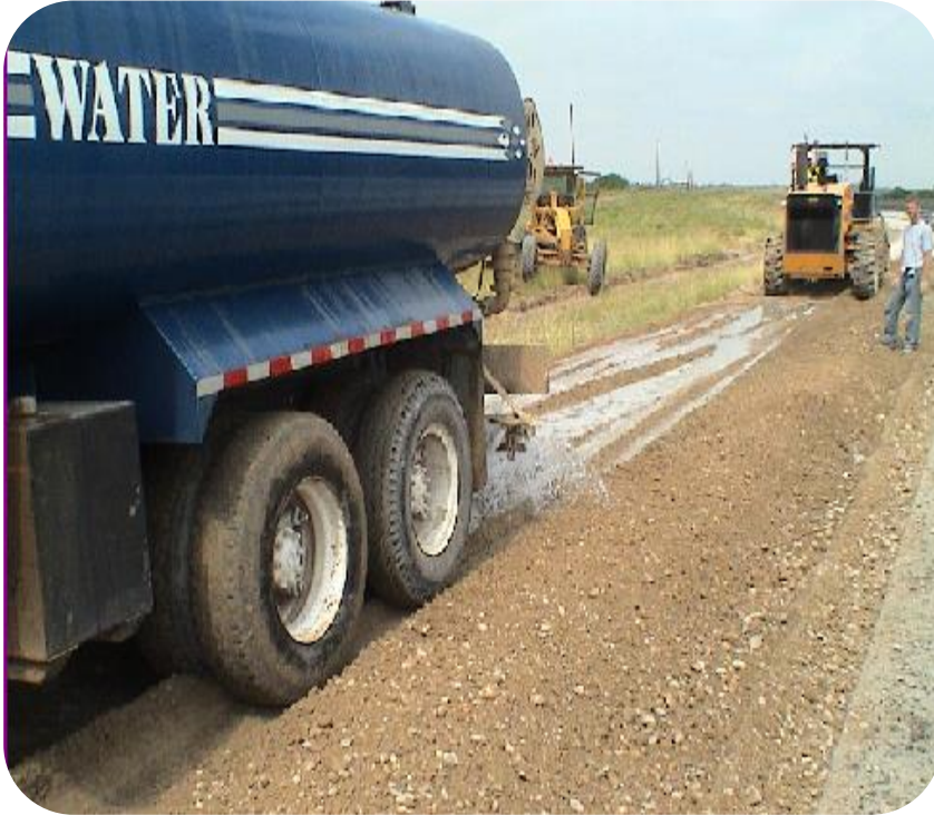
The soil is irrigated by a water tank to increase the natural water content
