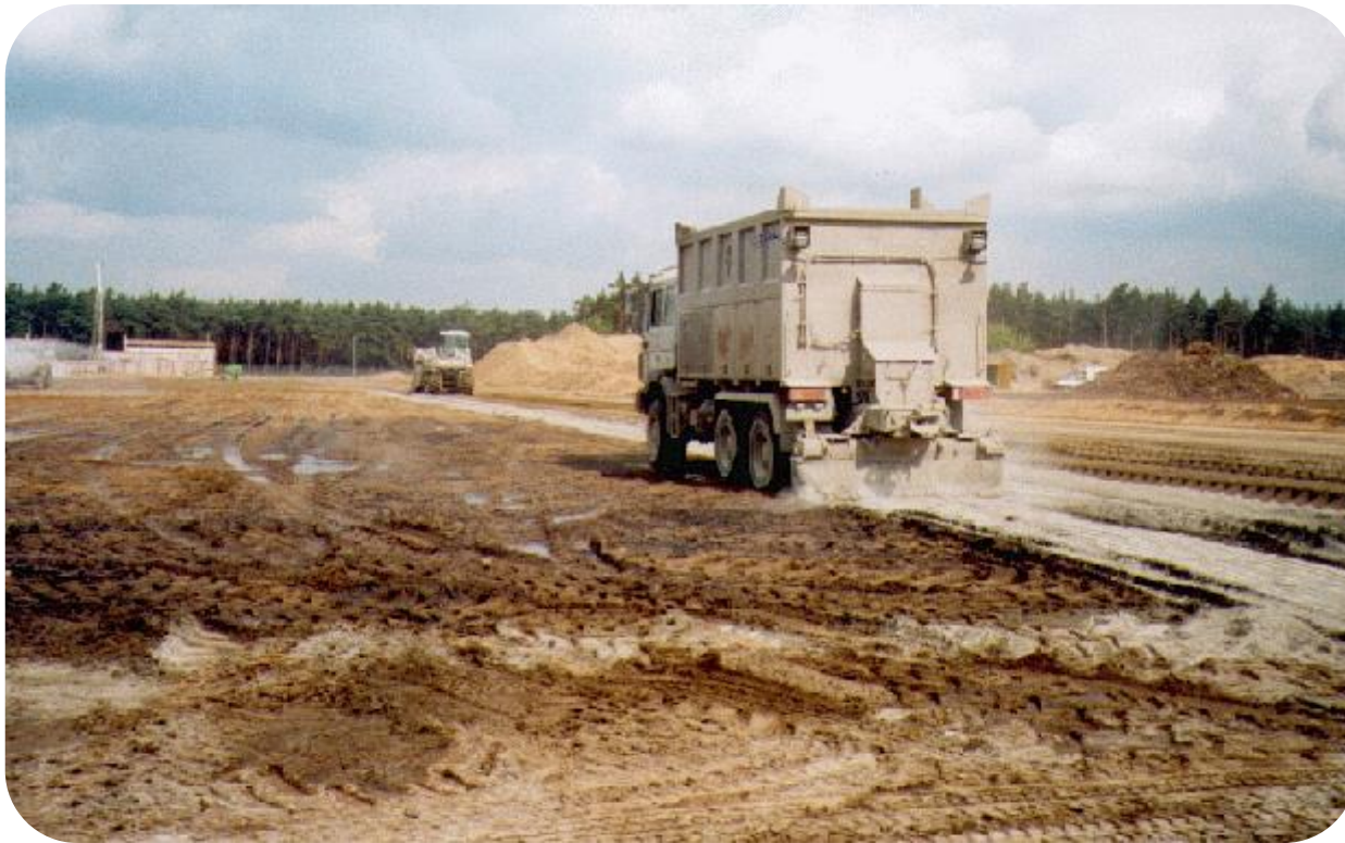
Cement spreader distributing the binding agent on the surface of stabilization layer
