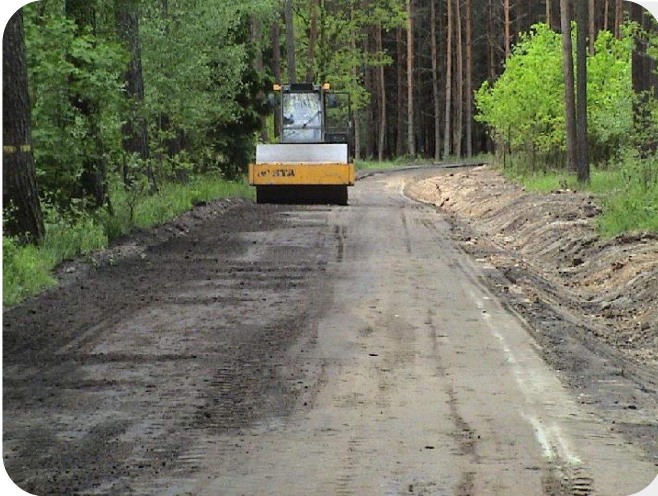
The steel jacket road roller compacting the ADDIMIX road base
