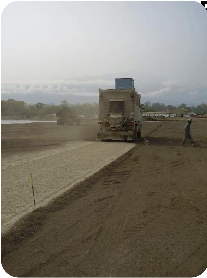
A cement spreader distributes the pure cement powder on top of the stabilization layer.
