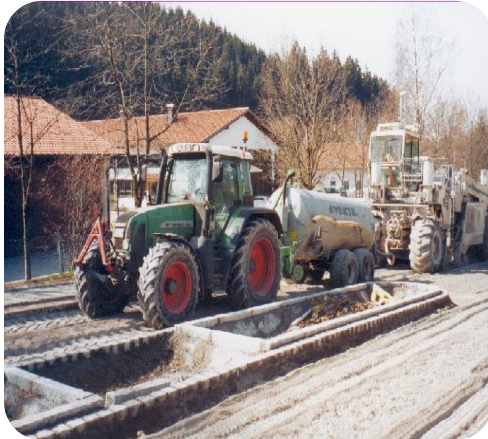
The WRS 2500 working during the mixing process with irrigation unit (tractor with water tank)
