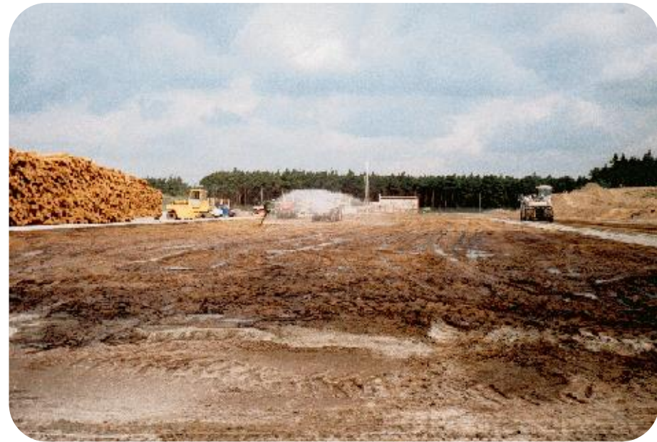
The sub grade is being irrigated because the dry weather conditions in summer has reduced the natural water content extremely
