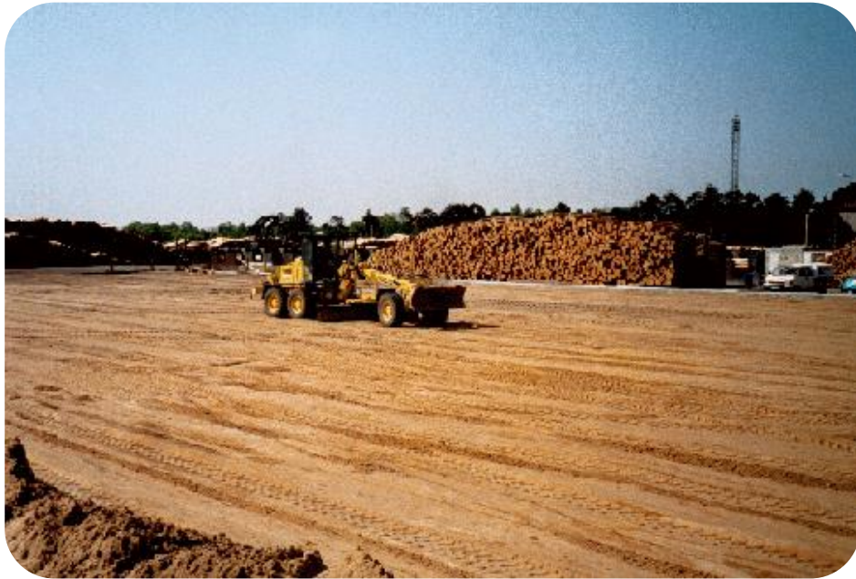
Subgrade leveling by grader
