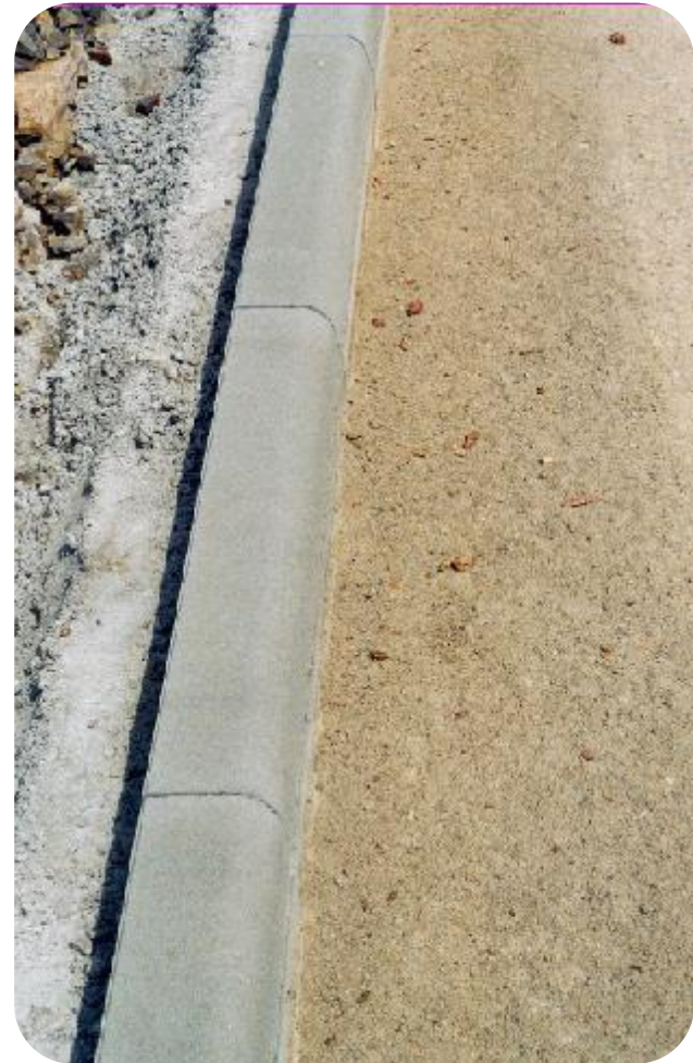
Contact area between curbstones and ADDIMIX road base
