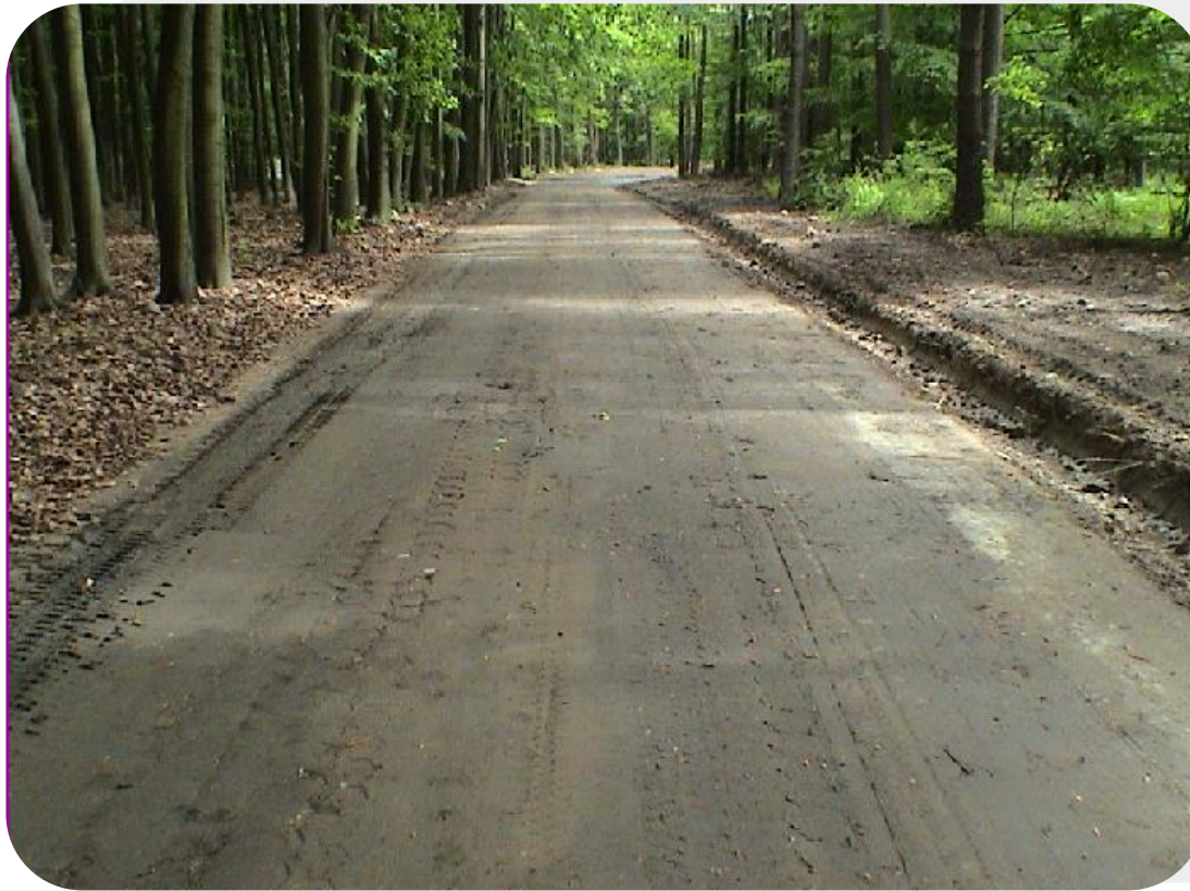
Fresh compacted ADDIMIX unpaved forest road
