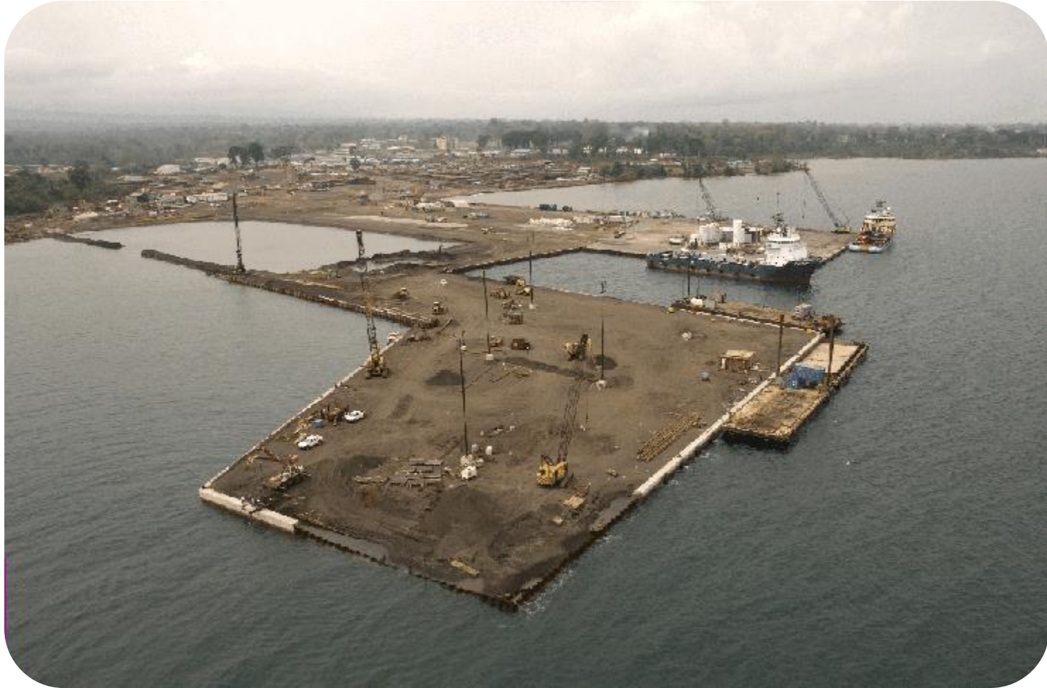
Land reclamation with dredged marine sand at the construction site in malabo
