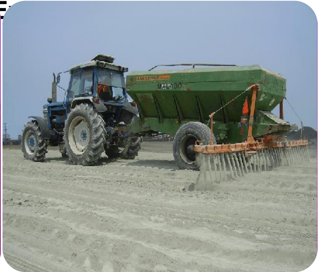
With an agricultural equipment ADDIMIX powder is spread on top of the cement layer.
