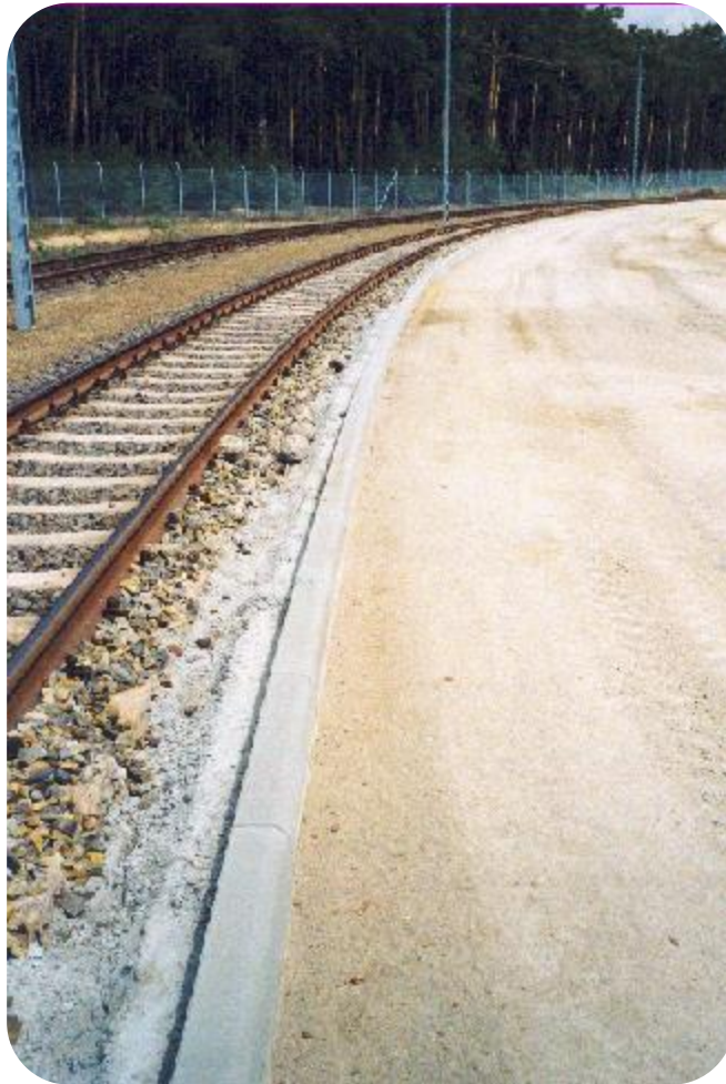
Contact area between curbstones and ADDIMIX road base
